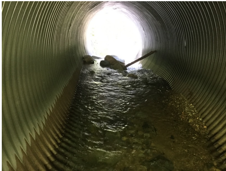
Material being transported into culvert
