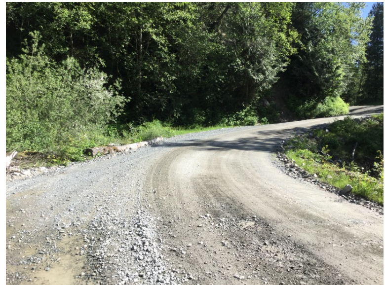
Approach from Right Bank when facing downstream
