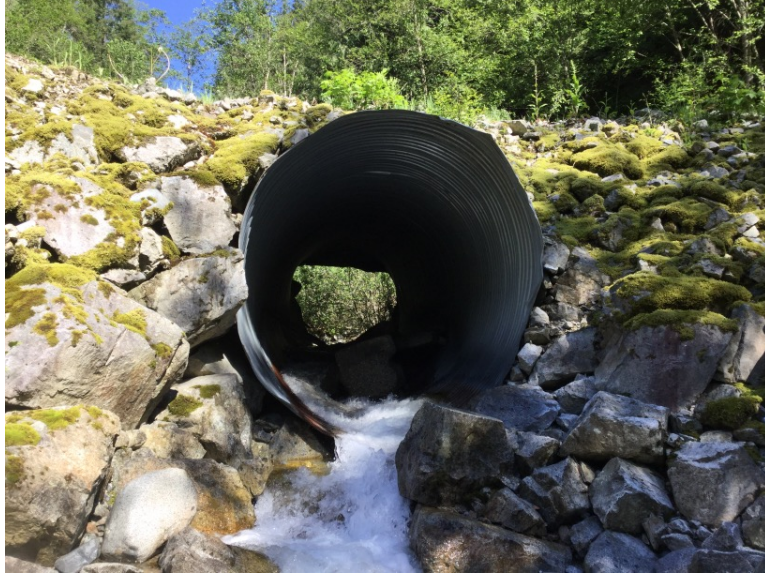
Culvert shape at outlet
